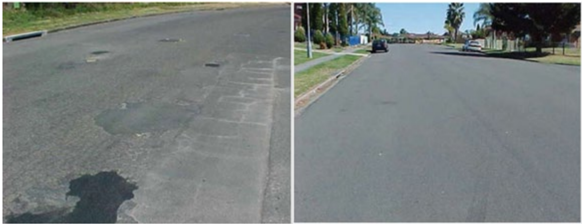
Figure 4. Road conditions before and seven years after reclamation with crushed concrete
